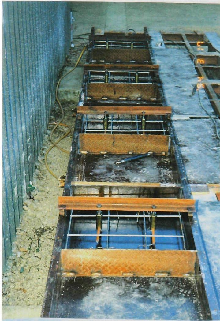
**Figure 5.5** Formwork and Reinforcement
