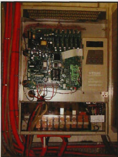
Figure 9: Internal of a VSD, with front cover removed
