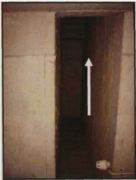
Figure 7: Separate supply air shaft
