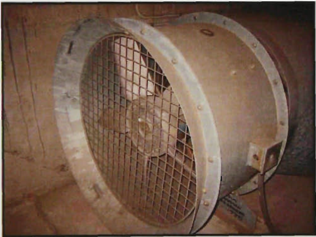
Figure 4: Axial Fan (example)
