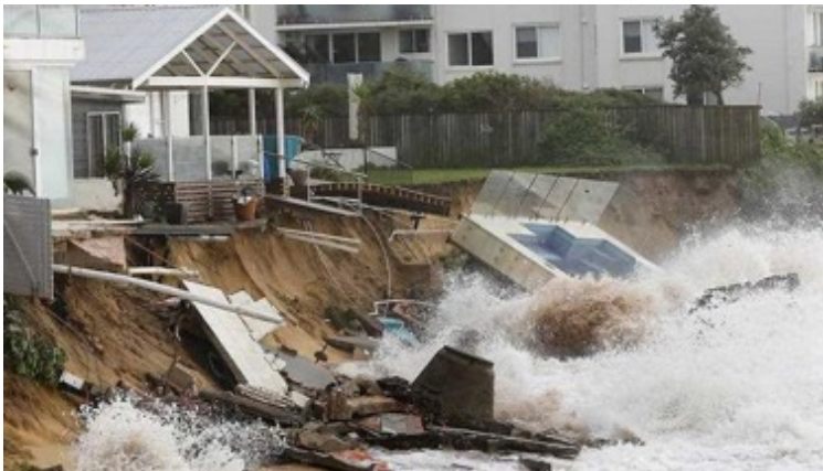
Figure 17 The veranda of a private house and backyard swimming pool fall into the ocean at Collaroy beach Sydney, after a storm and wave surge erodes the sand in June 2016 Photo sbs.com.au 7 th June 2016
