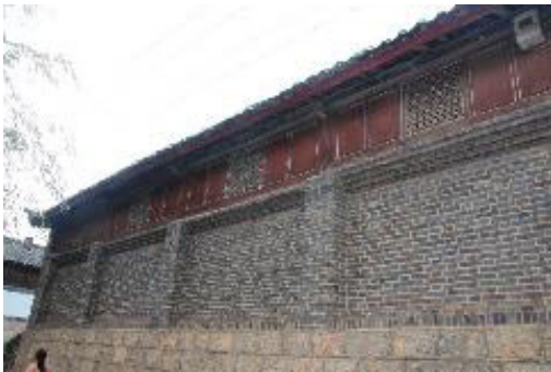
Figure 22. Walls constructed with three types of materials (photo by the first author)
