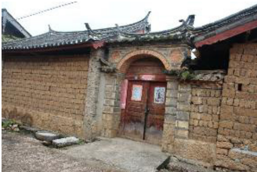
Figure 23. Buildings mainly constructed with adobe in a village of the Naxi (photo by the first author)
