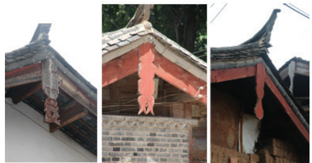
Figure 18. The board mimicking fish hung beneath the apex (photos by the first author)
