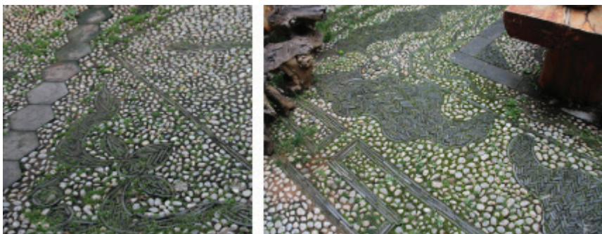
Figure 13. Paving with pebbles, tiles and bricks (photos by the first author)
