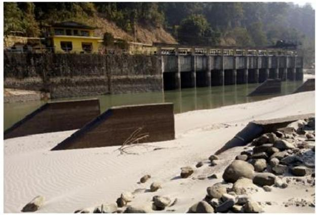
(c) Side-intake orifice with gates (gravity flow)
