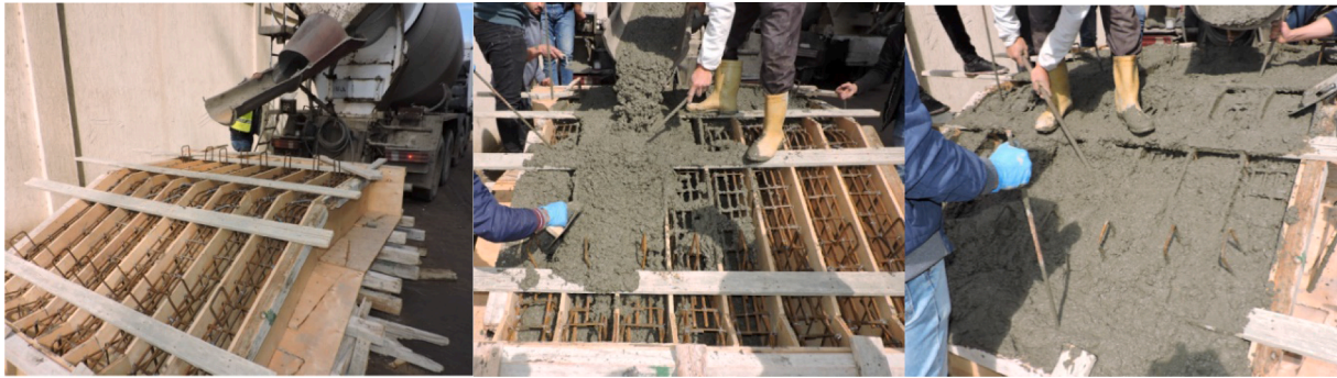
Fig. 3. Wooden formworks and field casting process.
