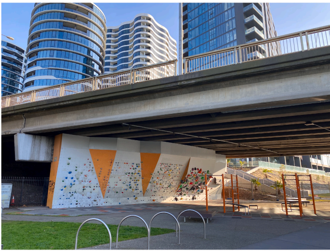
Fig. 3. Overview of arena for ecological literacy, Hopkins Street Bridge Bouldering Wall. Photo by first author.
