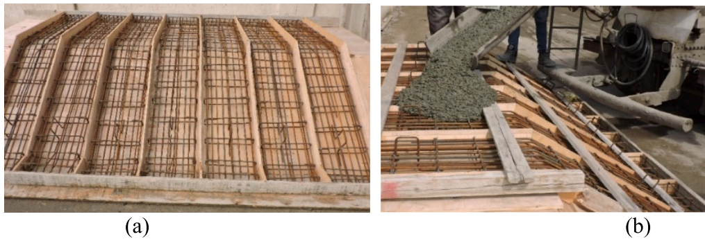
Fig. 6. Formworks and preparation: (a) wooden formworks; (b) during casting process.
