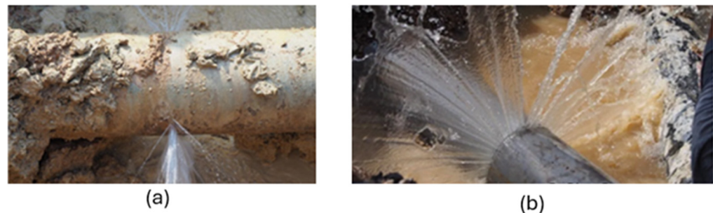
Figure 1. Showing (a) pipe leakage [3] and (b) pipe burst [4].
