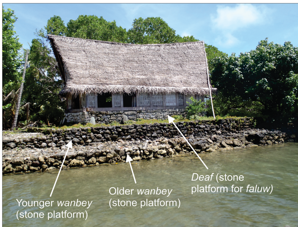
FIGURE 5 The faluw (men’s house) at Waalooy, Maap, Yap, showing how an extra stone platform (the younger wanbey ) was added to accommodate rising sea level, a TK-based adaptation to climate change.
