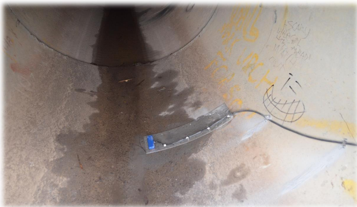
Figure 5-7- Flow meter sensor in the stormwater pipes
