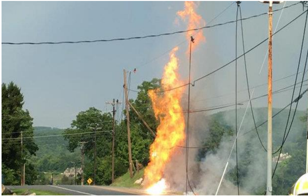
Fig 6.19: Fire creates due to HIF on trees [121]
