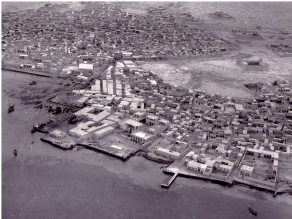
Figure 2-6 Aerial Image of Doha, 1947
