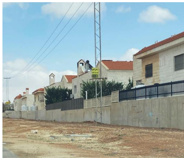
Fig. 3 The wall surrounding Al Andalucía development. Source The Author
