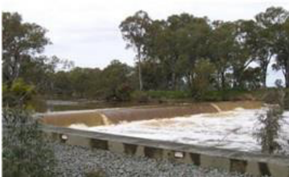
Figure A.3: Casey weir at lower flow showing fish ladder (Source: G-MW 2020)
