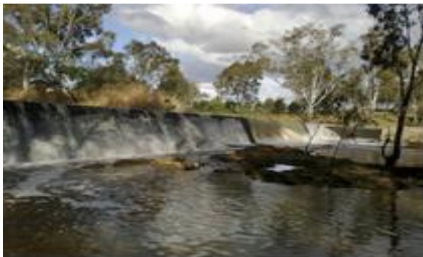
Figure A.5: Typical overtopped concrete weir, Broken River, Shepparton Victoria (Source: G-MW, 2020)
