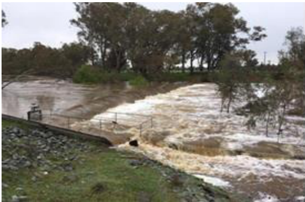
Figure A.2: Casey weir in flood (Source: G-MW, 2020)
