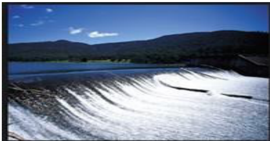
Figure A.4: A Pacific Hydro weir (Source: pacifichydro.com, 2020)
