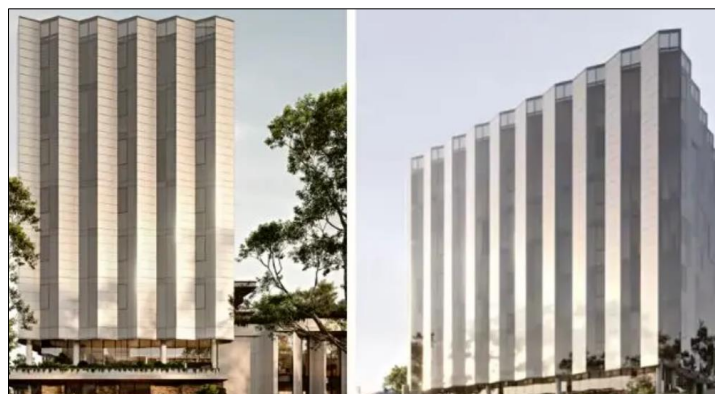
Figure 2-2. A modern building's entire exterior covered with solar panel skin
