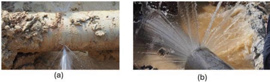
Figure 1.1: A typical (a) example of a pipe leakage (modified after R.S. Plumbing, 2024) and (b) example of a pipe burst (modified after Water Leak Detection, 2020).
